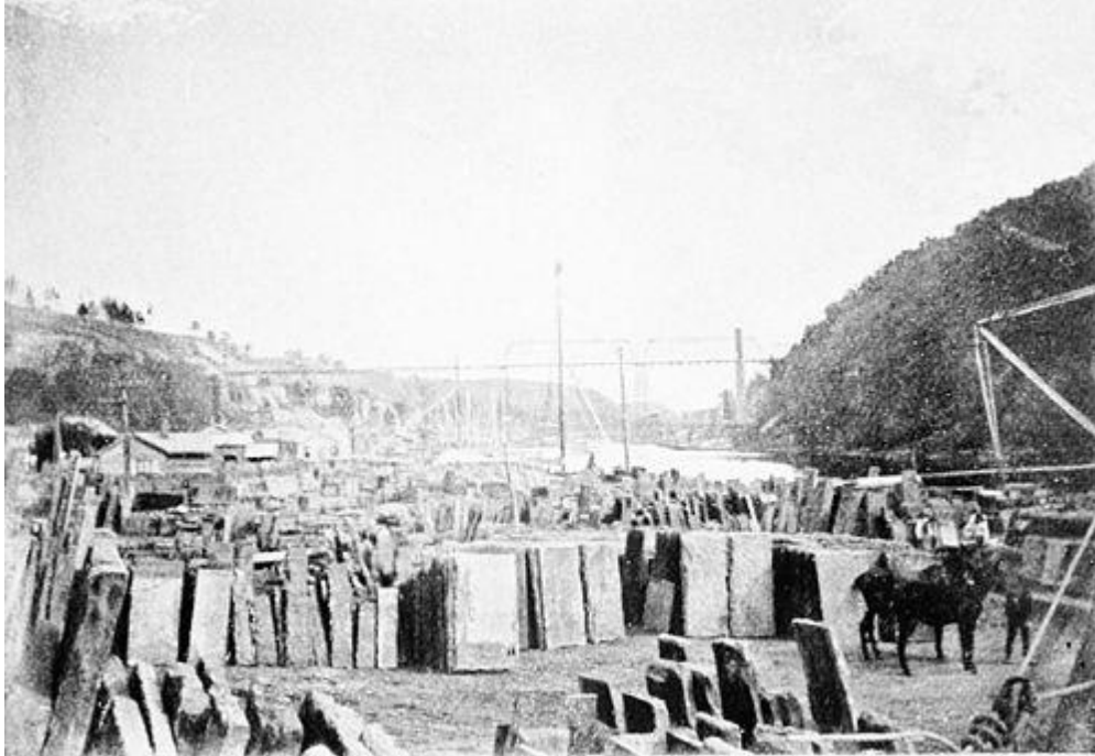
FIG. 4.—SHIPPING DOCK ON RONDOUT CREEK AT KINGSTON, N. Y.
