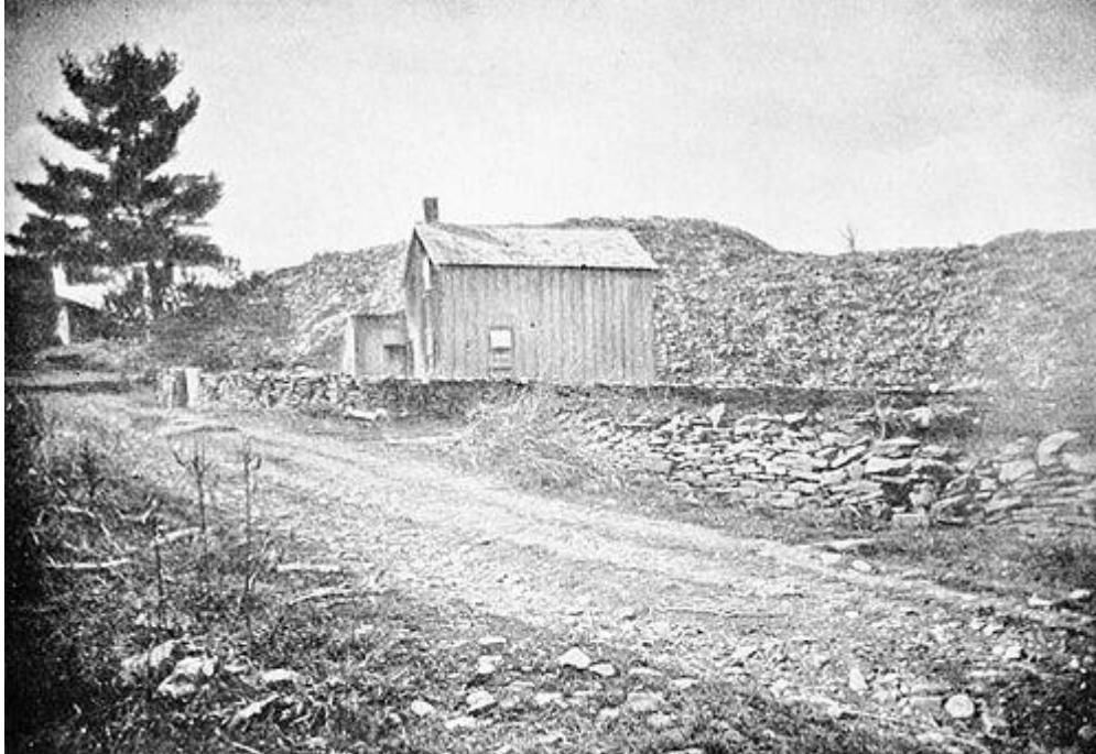
FIG. 3.—QUARRYMAN'S HOME WITH RUBBISH BANKS IN REAR, WEST HURLEY, N. Y.
